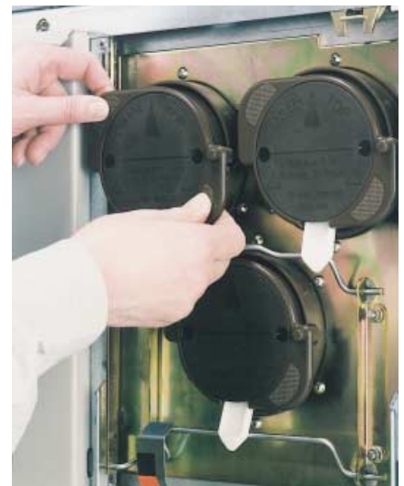
Fuse handle and all-pole tripping
