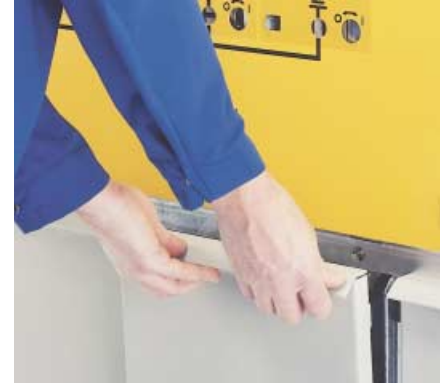
Removable cable compartment covers
